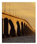
Completed in 1997, this fixed link across the Northumberland Strait used innovative design techniques including onshore construction, floating crane assembly, resulting in a 100-year service life. The design, build, finance, operate model replaced numerous ferry services operating between the two provinces. The Federal Government pays an yearly fee to Strait Crossing Inc., which in turn charges tolls to users under a 35-year agreement. *Photo credit: www.johnsylvester.com*
